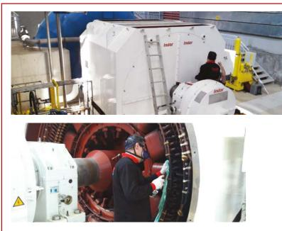
Our field failure detection field service is winding damage occured at 19 MVA generators due to water cooler puncture.
