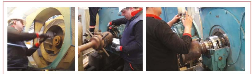
Shifting bed replacement and laser coupler adjustment of 2500 kW Atlas Copco compressor motor.
